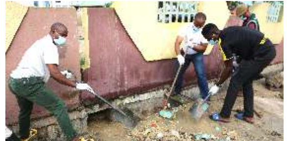
CU-CDIIC team cleaning drainage within the campus
